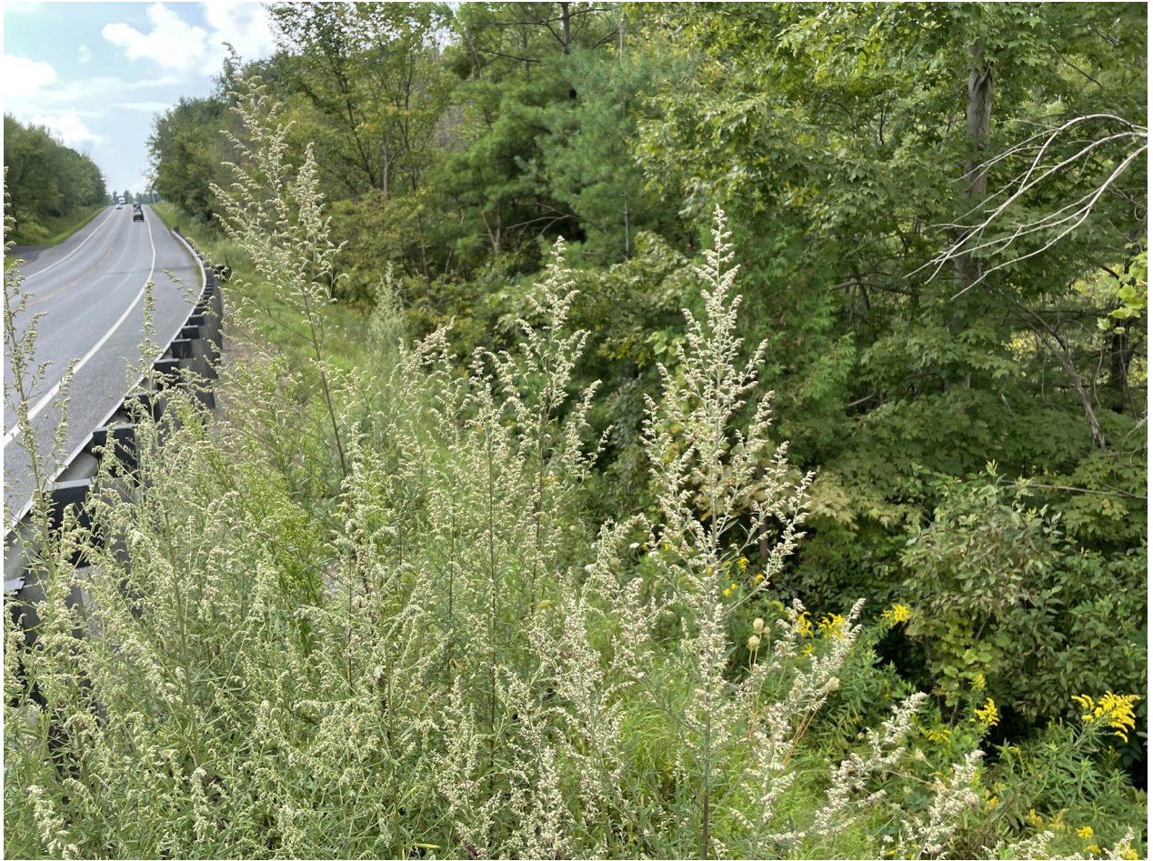
Figure 11. Southwestern bridge quadrant.
