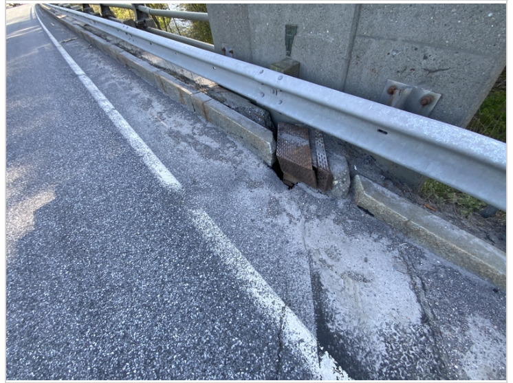
Abutment 1 upstream curb/joint end
