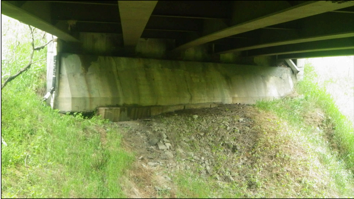
Appendix A 5: View of Abutment 2.
