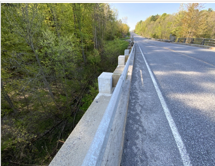
Upstream repaired rail
