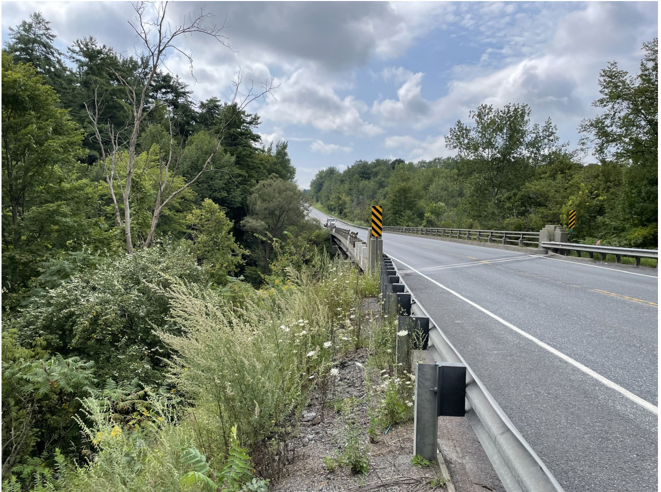
Figure 9. Northeastern bridge quadrant.
