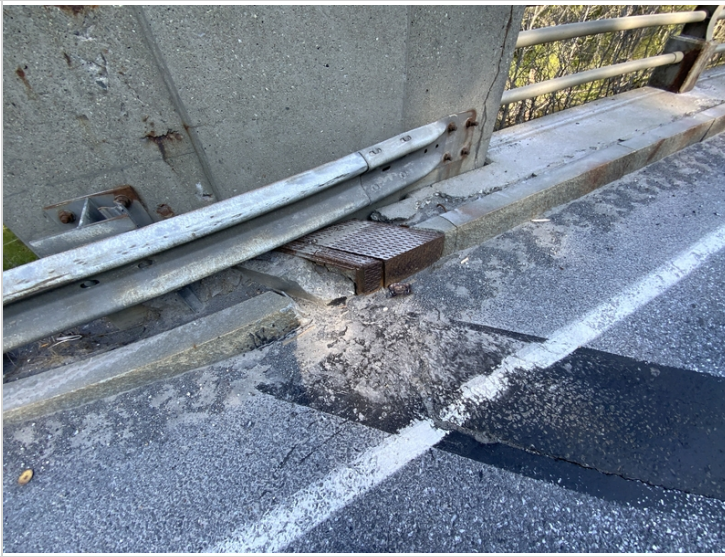
Abutment 1 downstream curb/joint end
