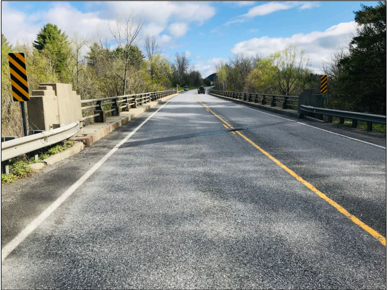
Appendix A 1: Approach of Bridge #138. The view is to the north.
