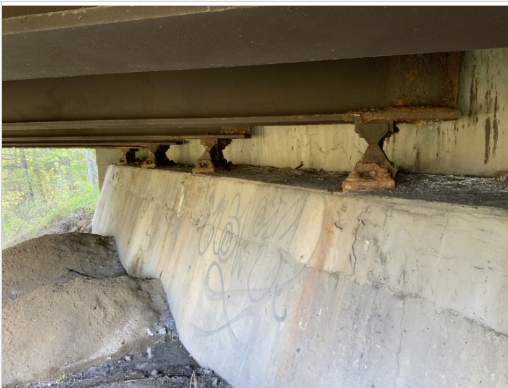
Abutment 1 bearings
