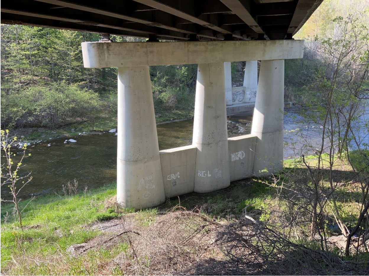
Appendix A 4: View of Pier 1.
