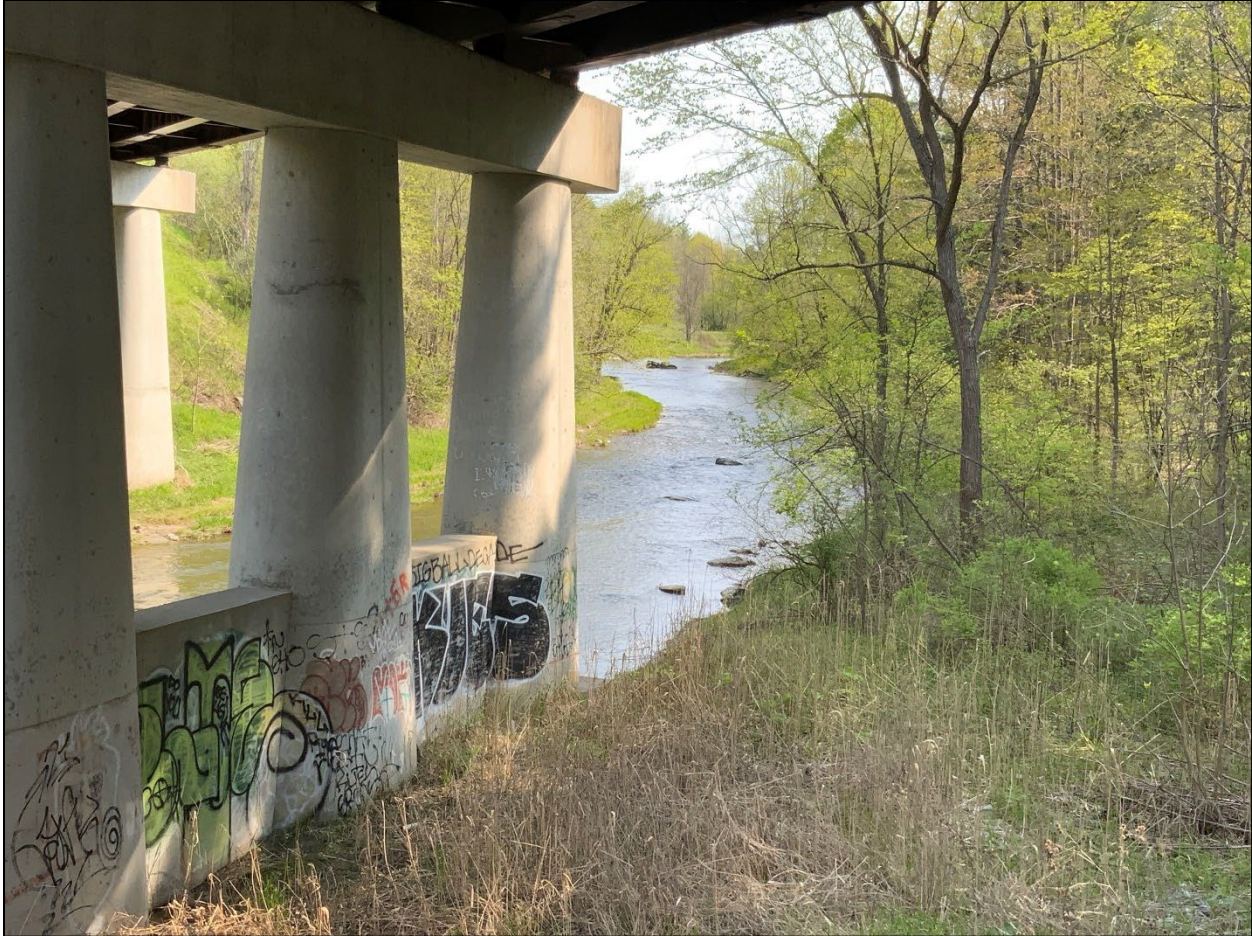
Appendix A 3: View of Pier 2.
