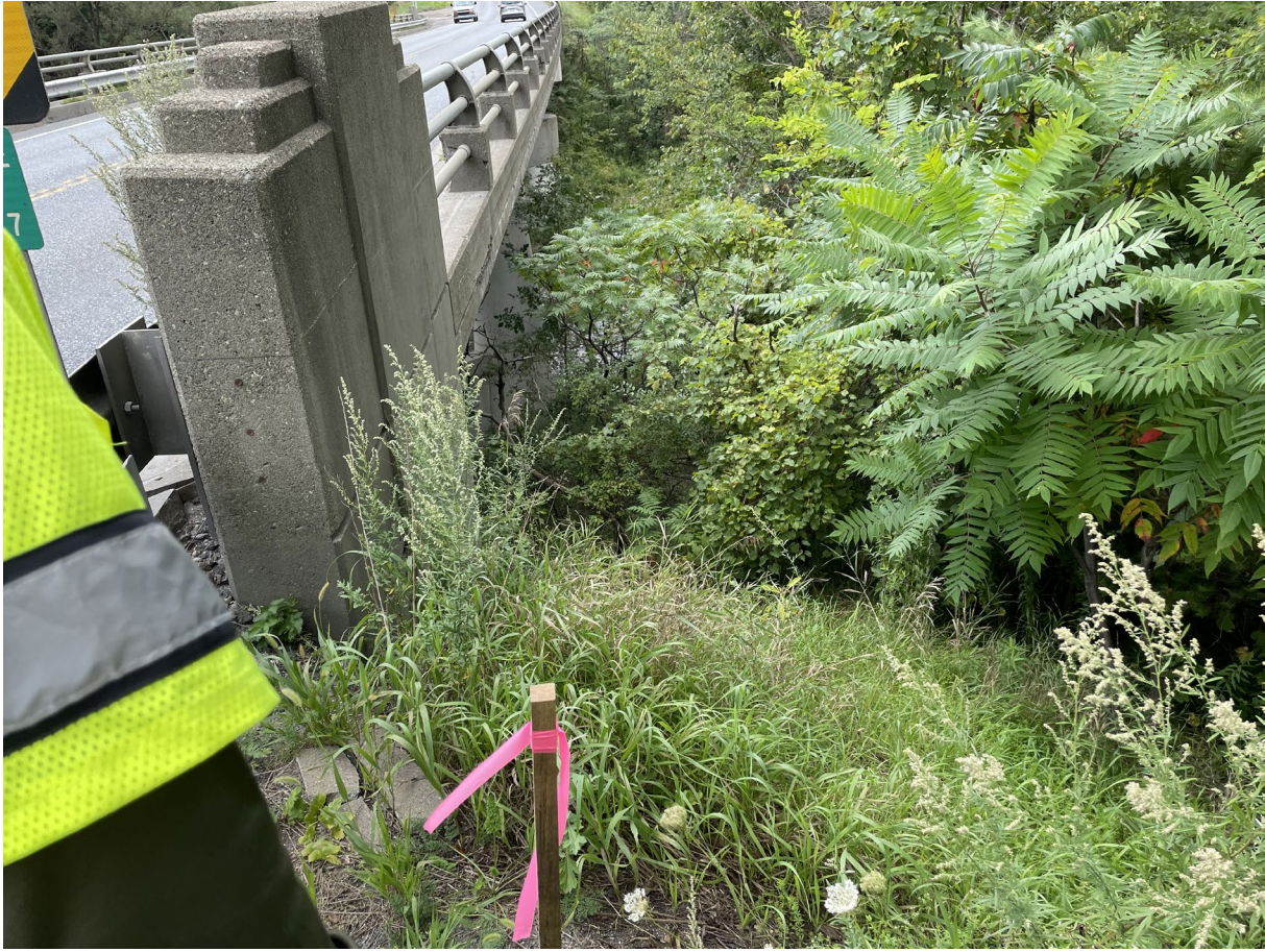
Figure 12. Southeastern bridge quadrant.
