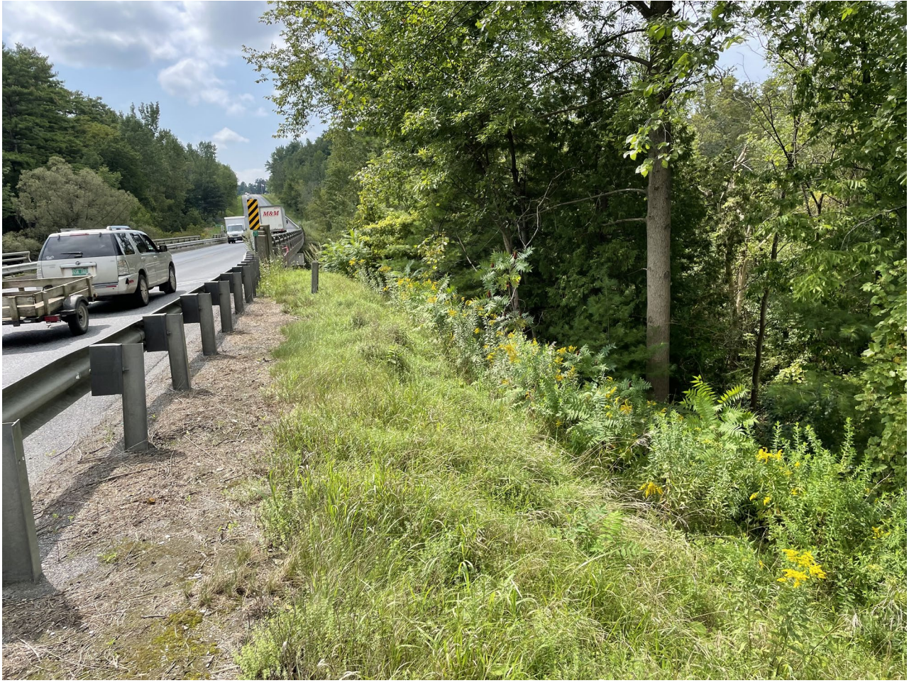
Figure 10. Northwestern bridge quadrant.
